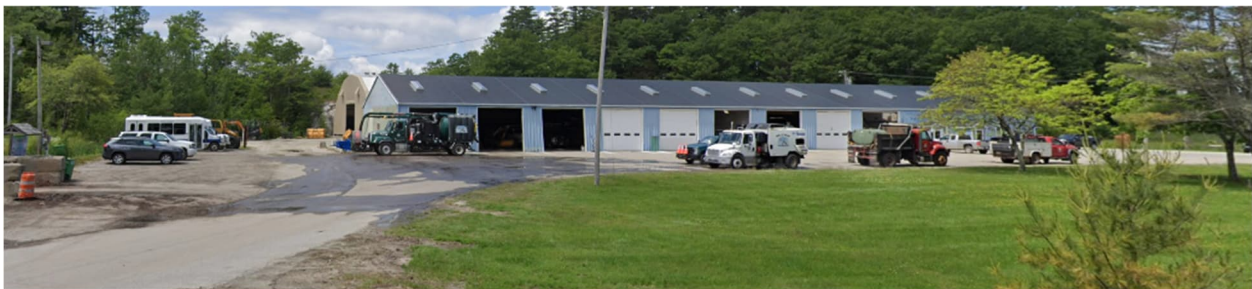
Figure 9 Bath Public Works Facility (Source: Google Maps)
